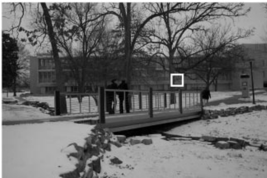
Fig. 1. The Smart Composite Bridge at the University of Missouri-Rolla. The location of the dedicated web camera is indicated on the building in the background.
