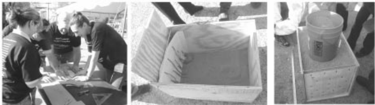
Fig. 4. The construction steps, and loading. (l to r) Cutting the paper, building the wall, loading the wall.
