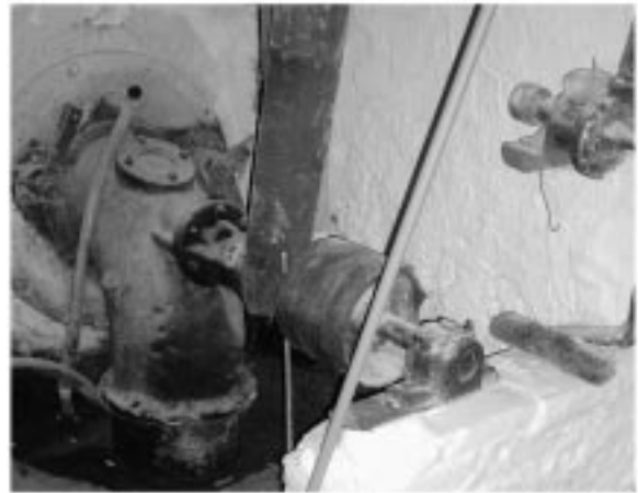
Fig. 7. Real state of centripetal turbine.
