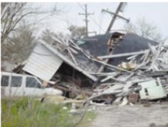
Fig. 5. Collapsed home in the Ninth Ward due to levee failure.
