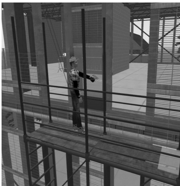
Fig. 5. Curtain wall installation.
