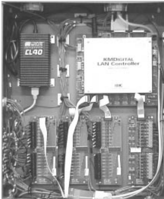
Fig. 2. A building automation system broadcasts solar collector data over the Internet.
