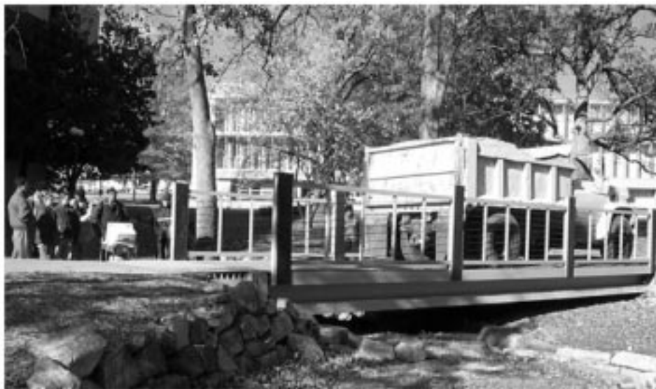
Fig. 3. Load test of the UMR smart composite bridge.
